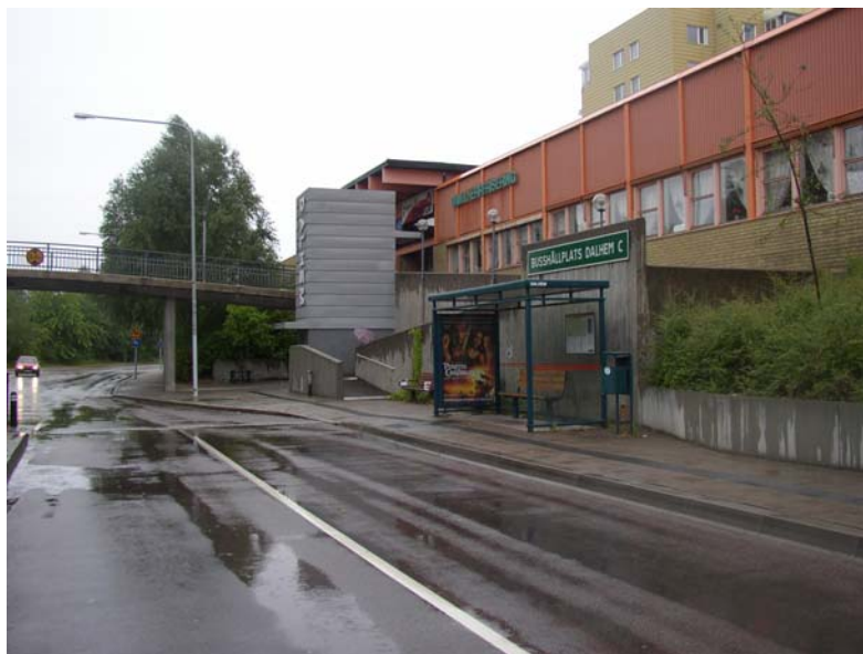
Hissinstallation i Dalhem
