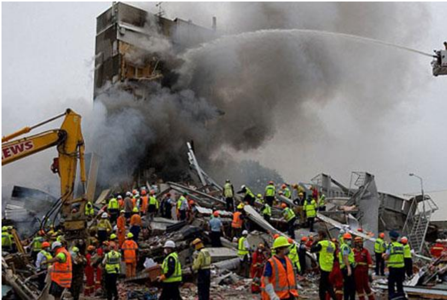
CTV building collapse
