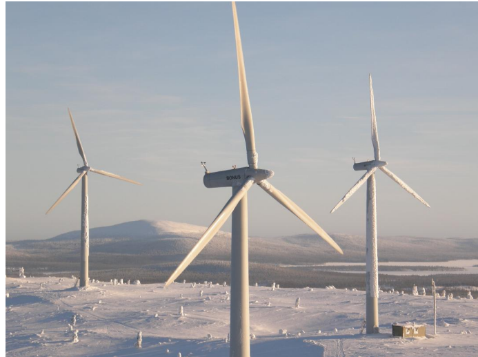
Figure 4. Example of an arctic wind farm from Finland (Olos 3 MW, 5 times 600 kW).
